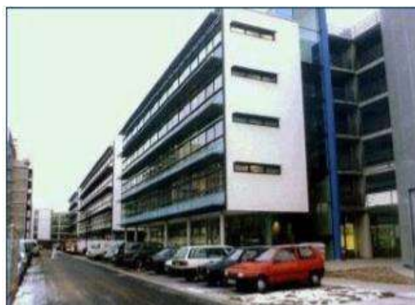
Figure 2: VilbelerWeg office building
